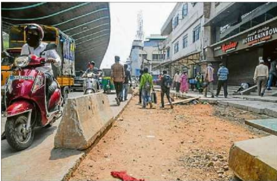
White-topping work underway at NR Road near KR Market. DH FILE/S K DINESH
