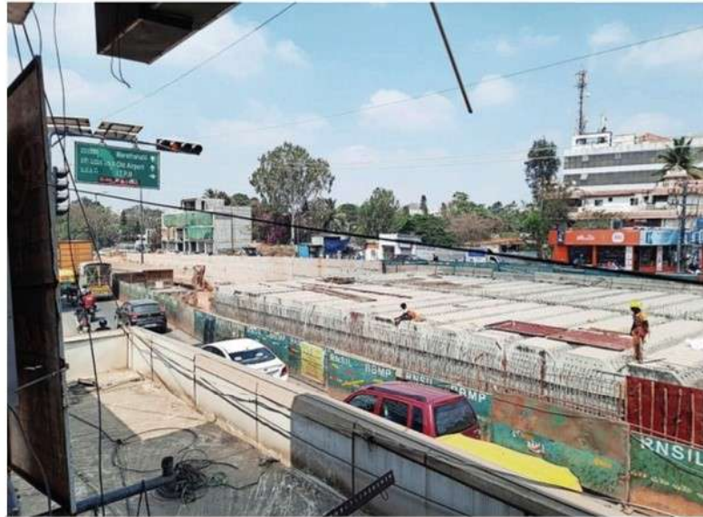
Work is going on at a steady pace on Kundalahalli underpass
