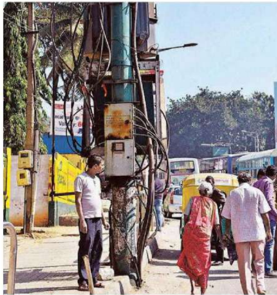
Pedestrians walk close to the electrical transformer on a footpath opposite Mysuru Road Satellite Bus Station in Bengaluru. *FILE PHOTO
